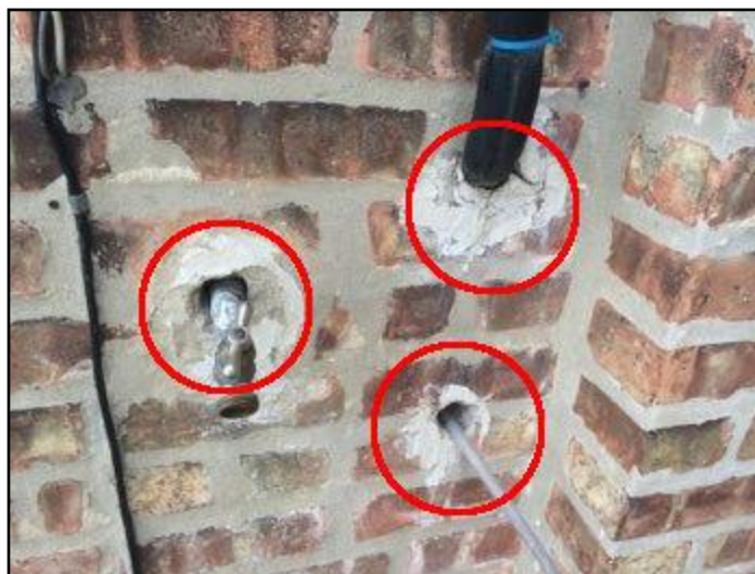
21. Caulking deteriorated
