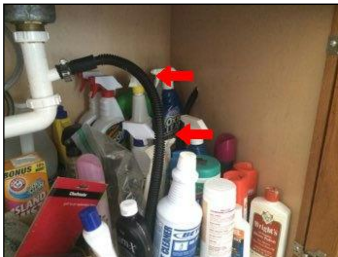
75. Backflow prevention missing
