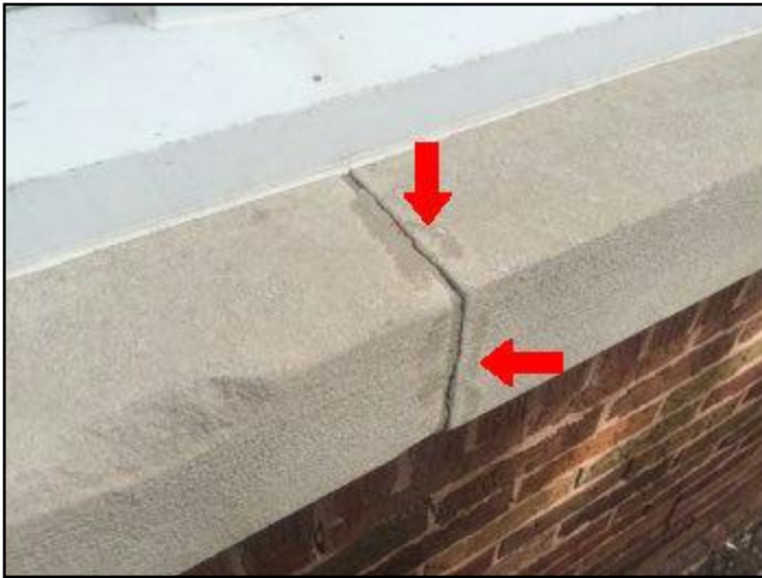
17. Caulking missing at window sill(s)
