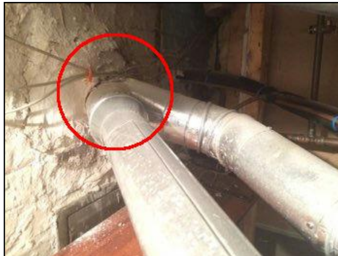
49. Appliance vents into chimney flue
