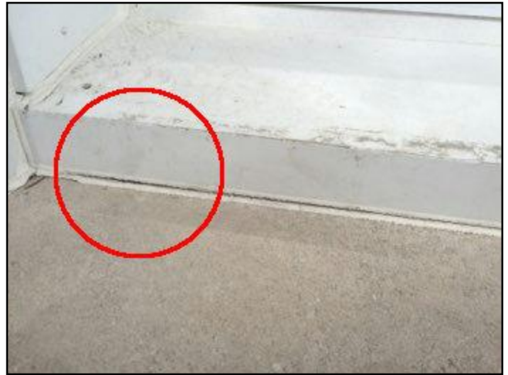
18. Caulking deteriorated at various windows
