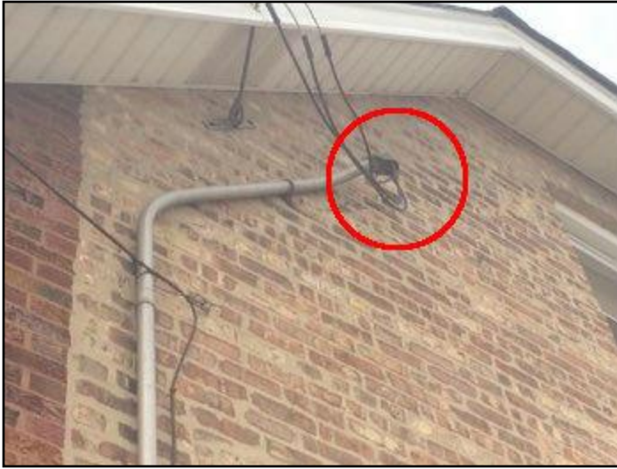
33. Service entrance pulled away from wall
