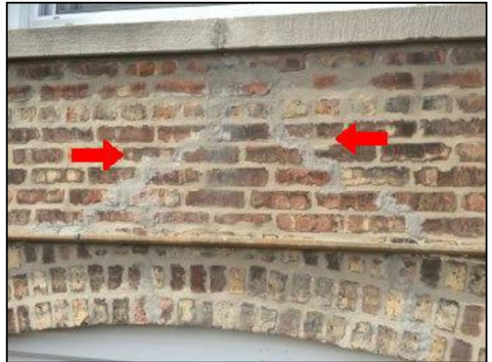
15. Cracked east wall under window sill
