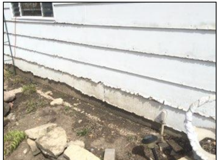
27. Rot at exterior wall
