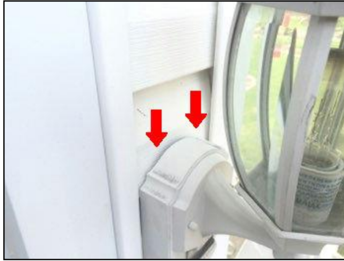
36. Missing caulking at exterior light
