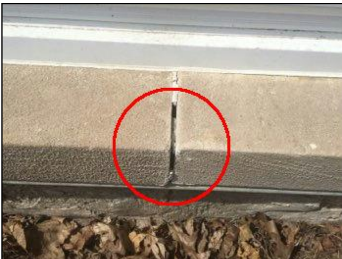
19. Caulking missing at window sill(s)
