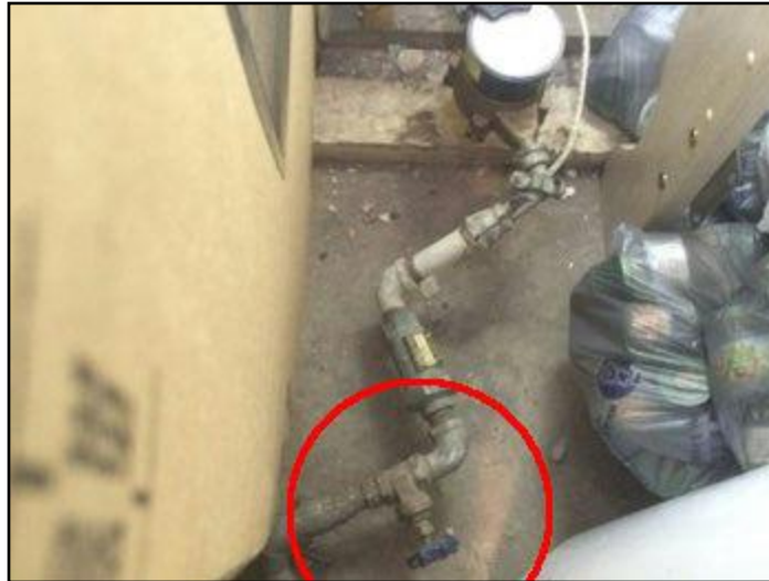
59. Basement main water shut off
