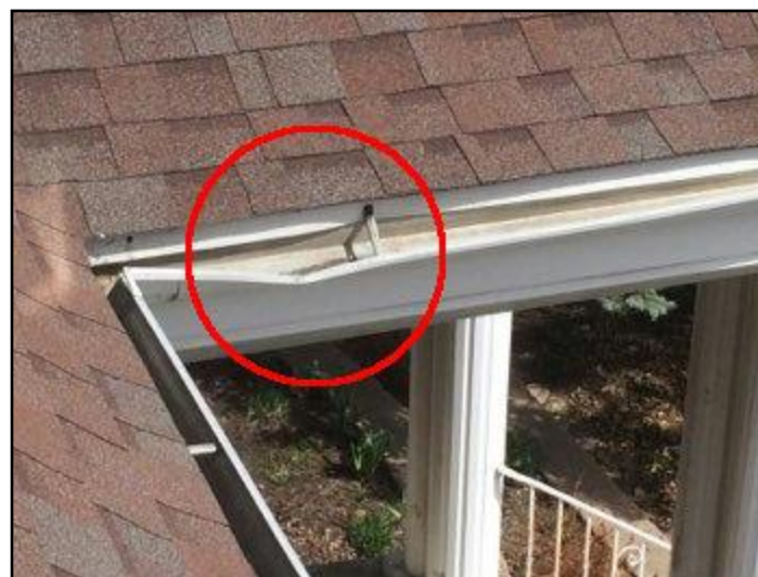
12. Damaged gutter w/ improper slope
