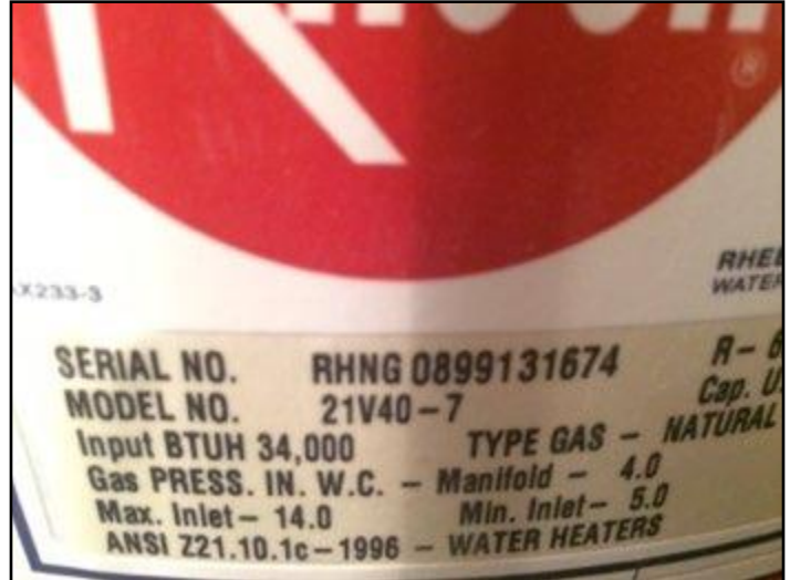
62. Rheem water heater ratings tag
