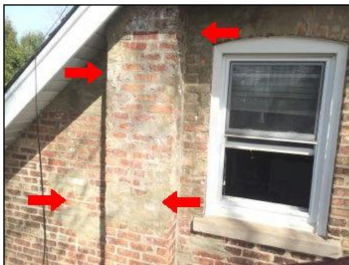
47. Parging repairs
