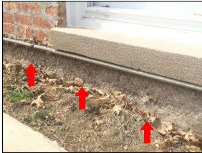
29. Spalling and crumbling cement at foundation
