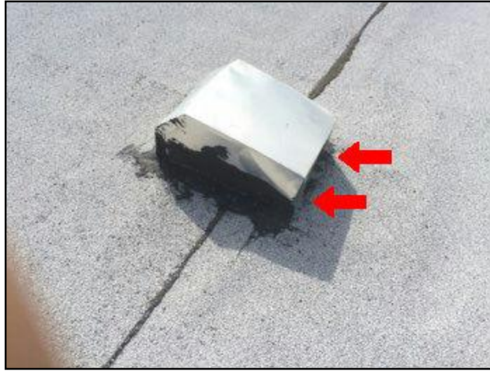
13. Improper flashing
