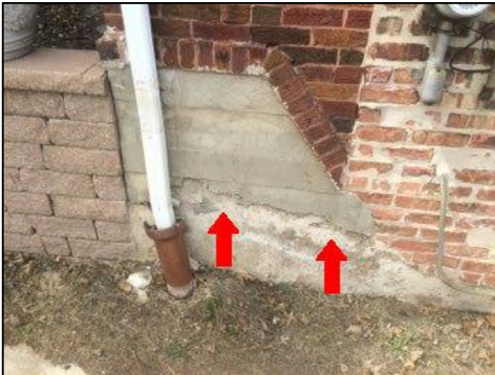
30. Parging damaged
