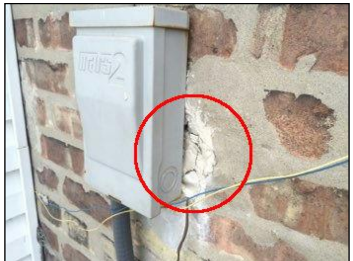
20. Caulking deteriorated at A/C disconnect
