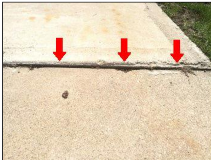
24. Uneven (trip hazard) at driveway
